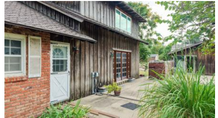
Detached garage/carriage house exterior
