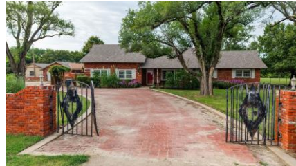
Front elevation from the entry gate
