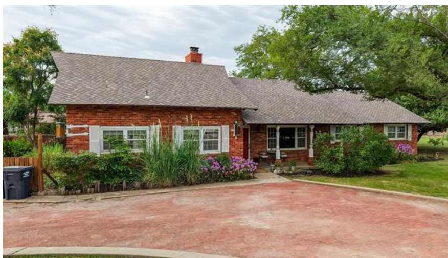
Front exterior view of the subject property, a brick ranch home on a 2.08± acre corner lot.
