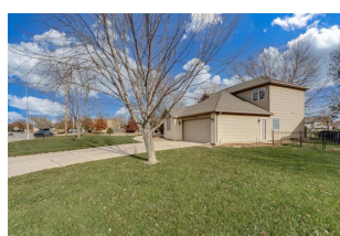
Side Of Structure
