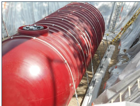
Tank being anchored to concrete deadman (right side, bottom of the basin) using straps
