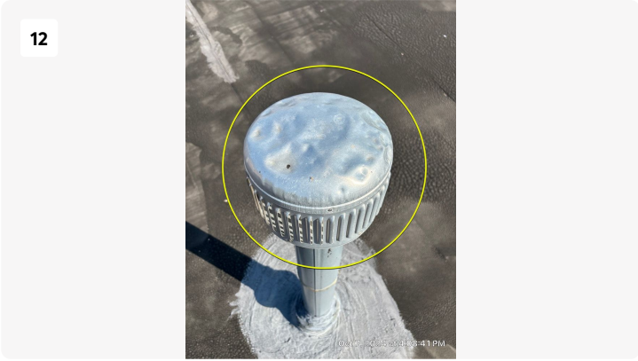
Soft metal hail damage.
