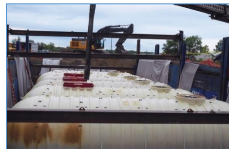
Tank installation excavation showing shoring and bracing
