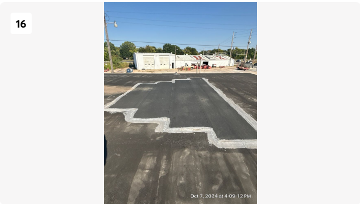
Large patch work completed.
