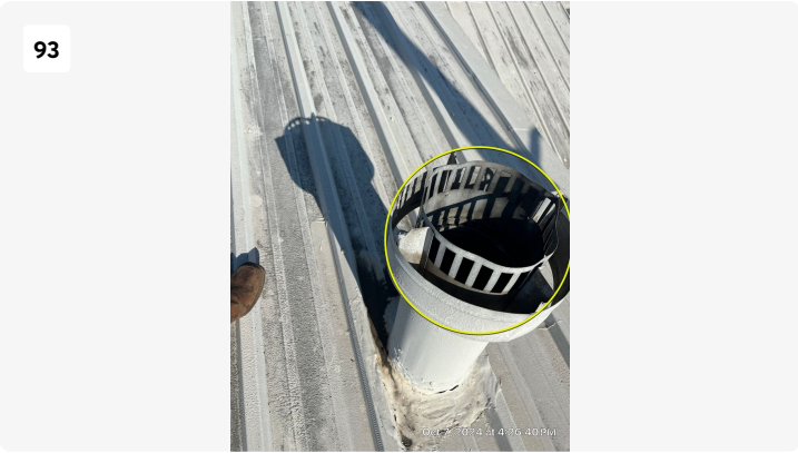
Missing vent cap.
