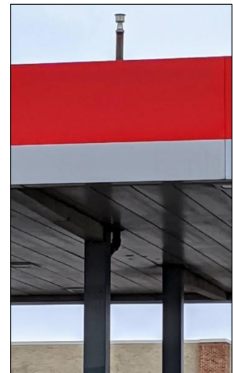
Example of vent line positioned above awning
