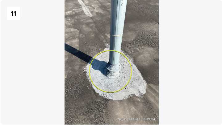
Penetration needs re worked.
