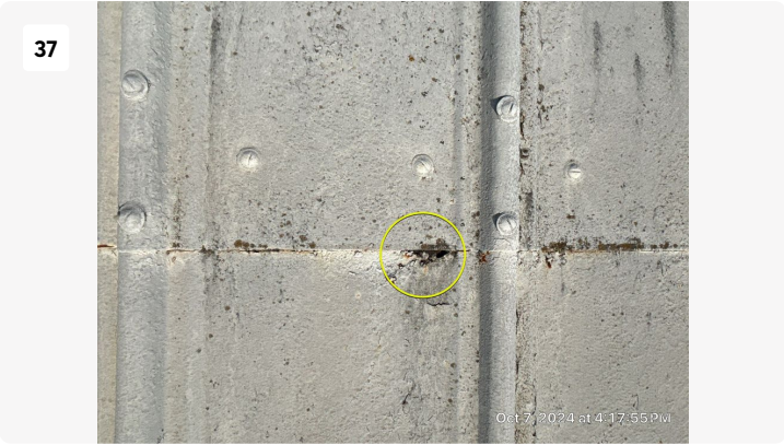
Pin hole in metal panel.
