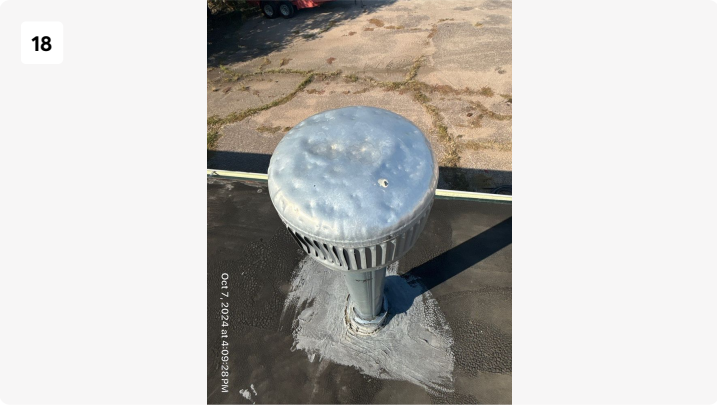
Soft metal hail damage.
