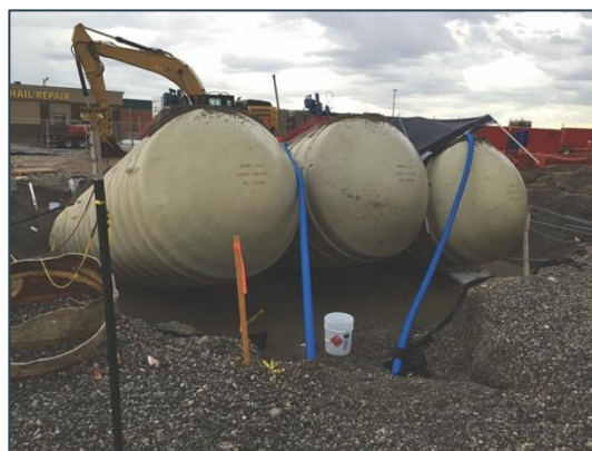
Tanks floating due to stormwater intrusion during installation before securing anchoring system
