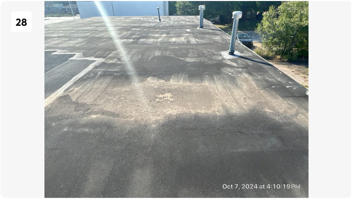
Soft spot, roof system and decking compromised.
