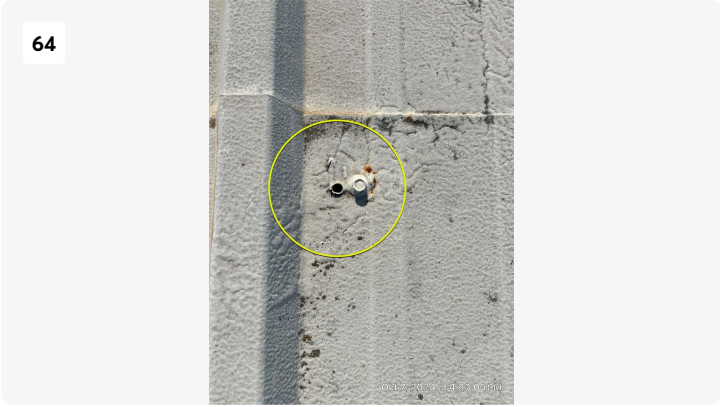
Missing screw hole on upper roof.
