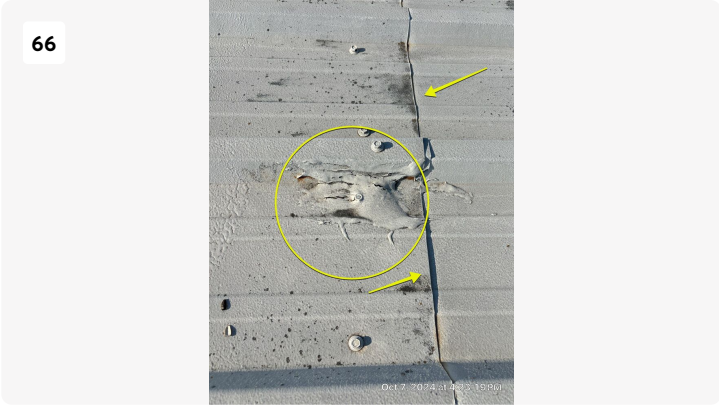
Metal panels showing gaps in overlap and silicone over fasteners.
