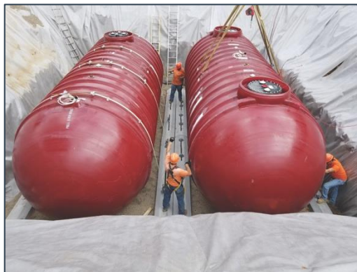
Two USTs mid-installation
