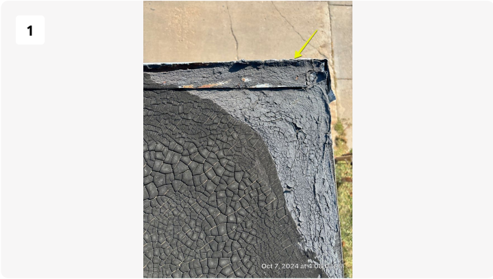
Metal edge pulling away from the roof.
