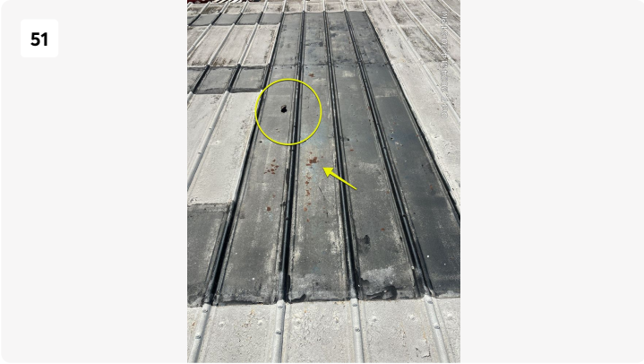
Hole in metal panel and rust.
