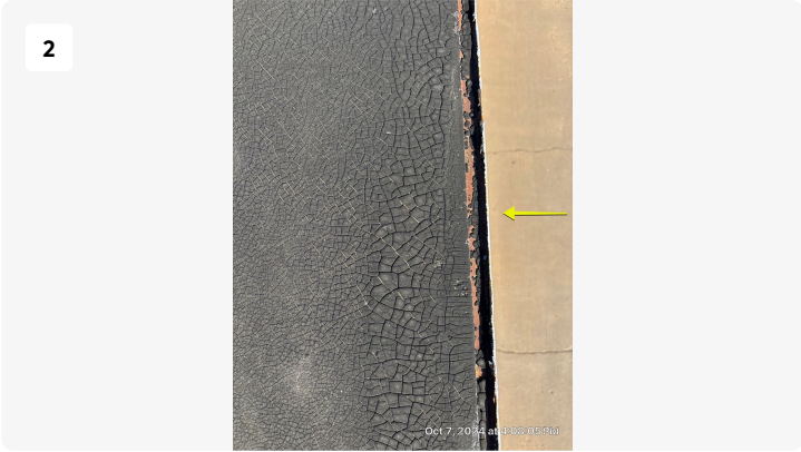
Metal edge pulling away from the roof.
