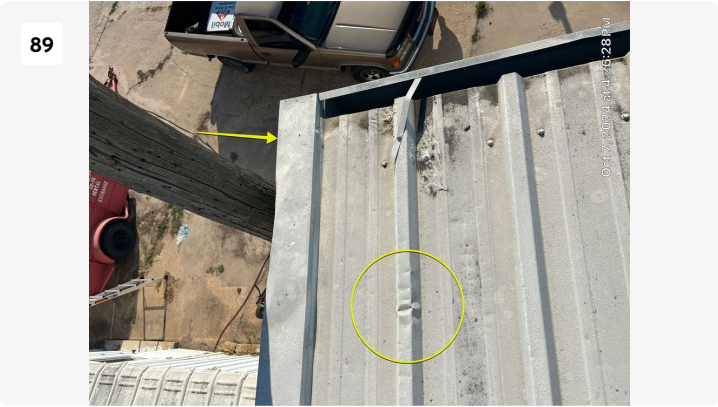
Soft metal damage and r panel damage.
