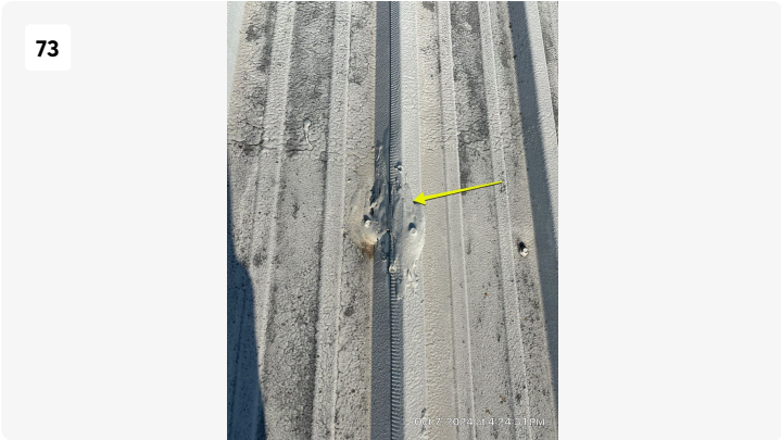
Metal rib damage.
