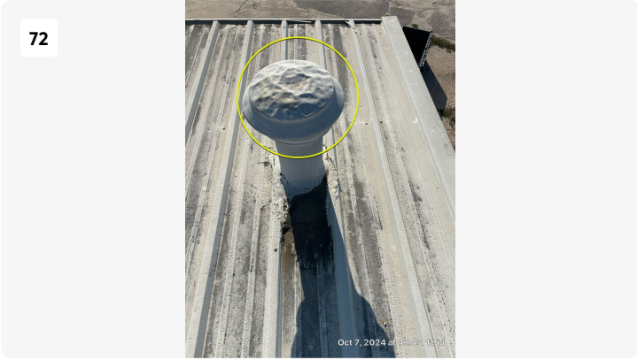
Soft metal damage.
