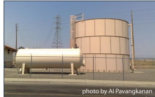
A horizontal storage tank (left) and a field-constructed tank (right)
