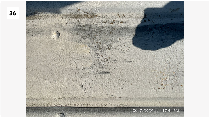
Rust and cracked coating.
