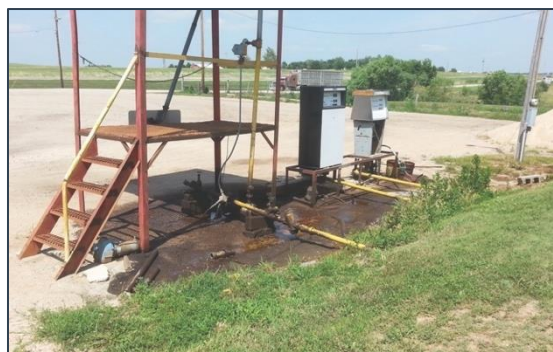
Product on the ground, indicating a spill or release
