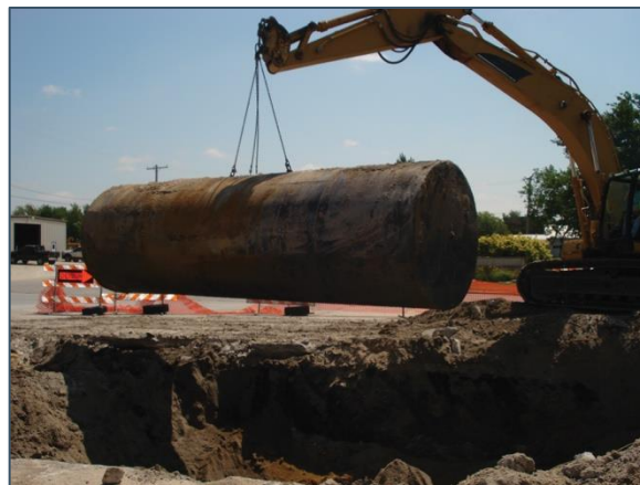
UST being removed from service
