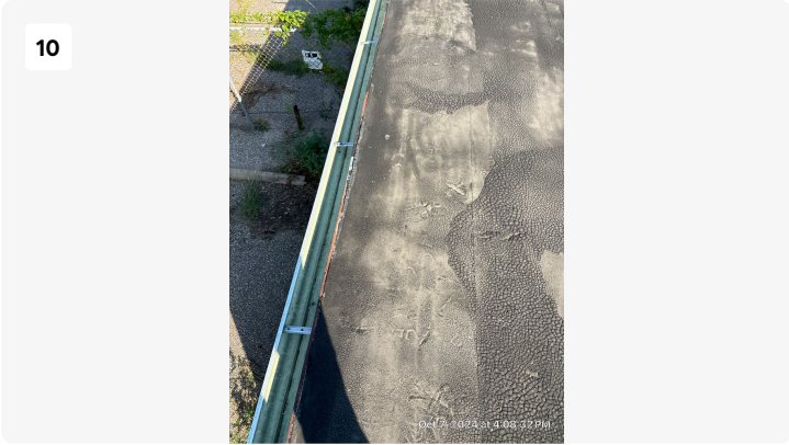
Metal edge rusted, field membrane alligatoring.
