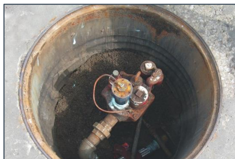
Example of an STP sump
