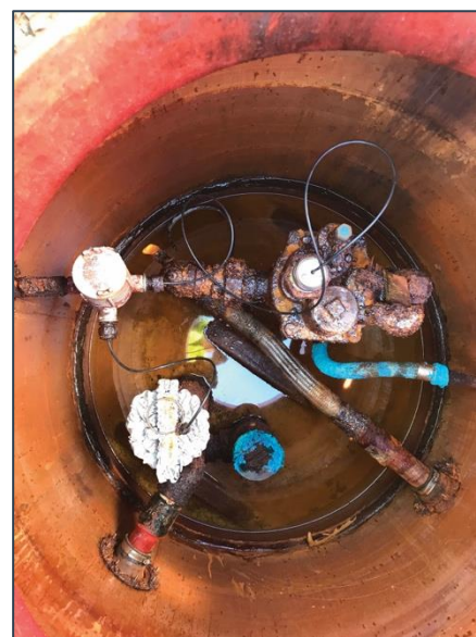
Example of corrosion due to bacterial growth (image courtesy of Ed Haselwood)
