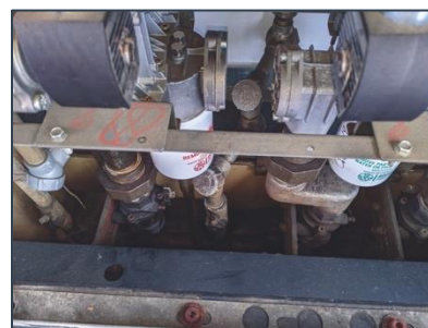
Example of under dispenser containment, or UDC
