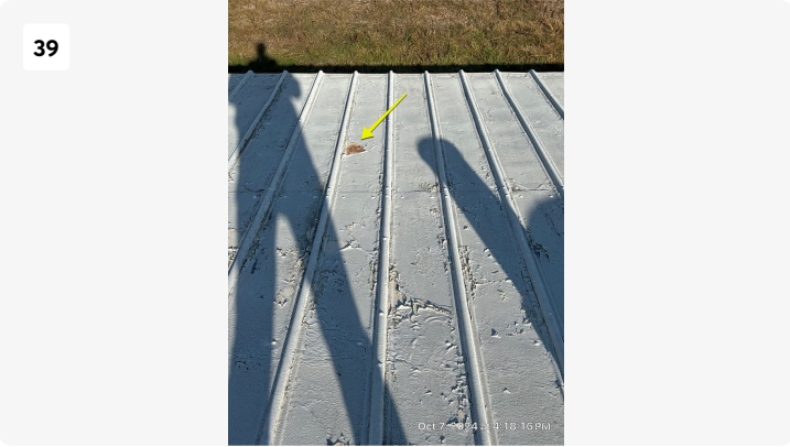
Failing coating and rust showing.
