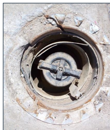
Example of a damaged spill bucket
