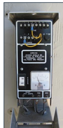
Example of a rectifier, which is part of an impressed current cathodic protection system
