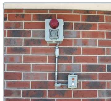
Example of an overfill alarm with attached emergency shutoff
