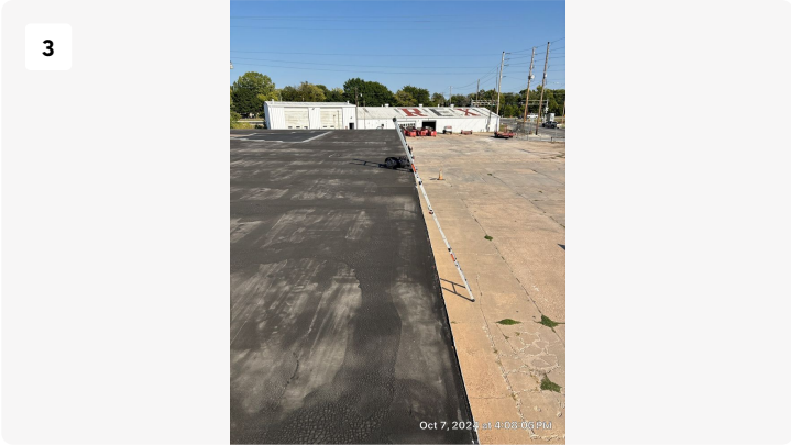
Overview - roof is scrimmed out, and losing the overall MIL or thickness of the asphalt roof.
