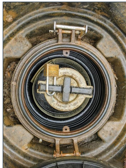
Example of a spill bucket with label inside
