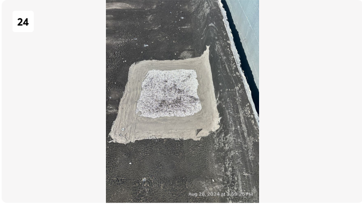
Deleted penetration stripped in with modified cap sheet and 3 coursed.
