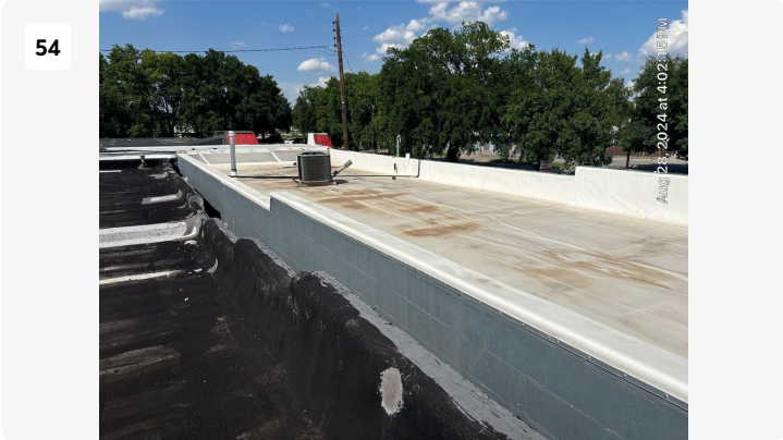
Roof next door has been roofed, and wall flashing terminated up and over the wall surface with termination bar. Good example of what 1028 could possibly look like.
