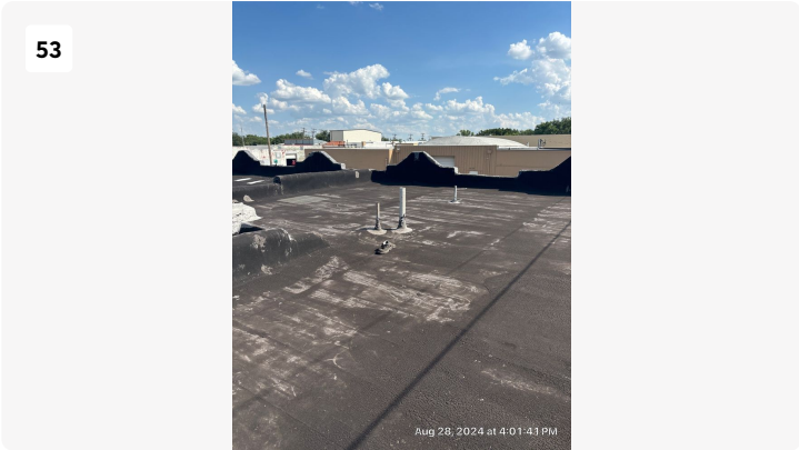
Project: 27835 1028 East Harry Date: 8/28/2024, 4:01pm Creator: Evan Smith
