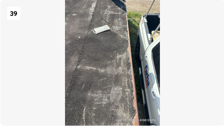
Project: 27835 1028 East Harry Date: 8/28/2024, 4:00pm Creator: Evan Smith
