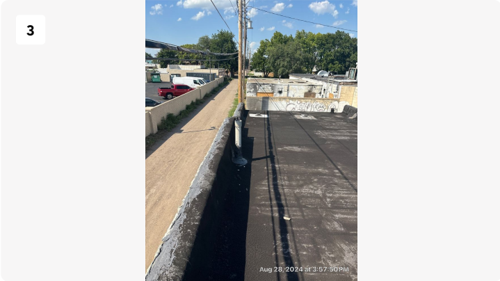
Overview, southwest elevation.
