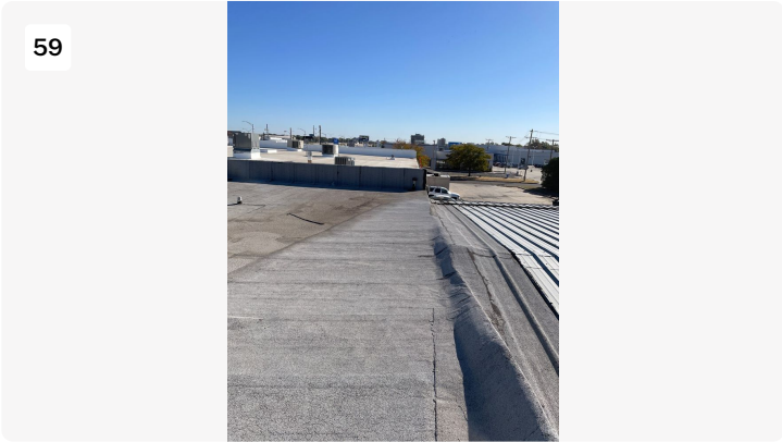
South wall on mod bit roof.
