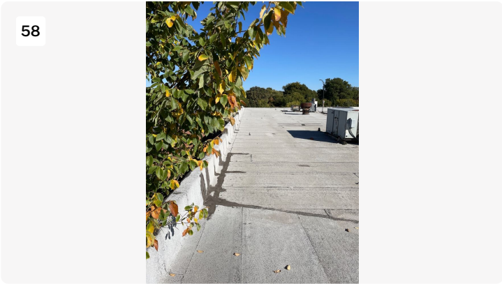
West wall on mod bit roof.
