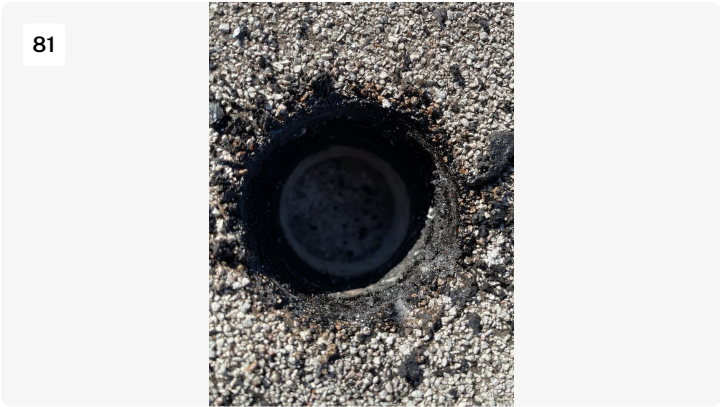
Core sample on mod bit roof; shows deck type & roof makeup.
