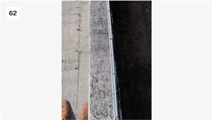
Overview of termination bar.
