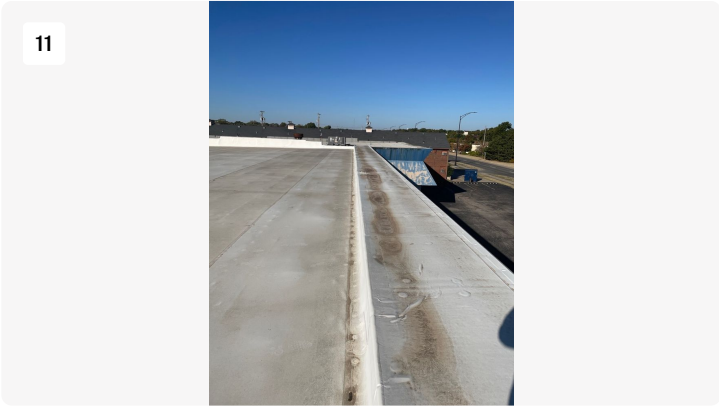
Overview of north TPO wall.
