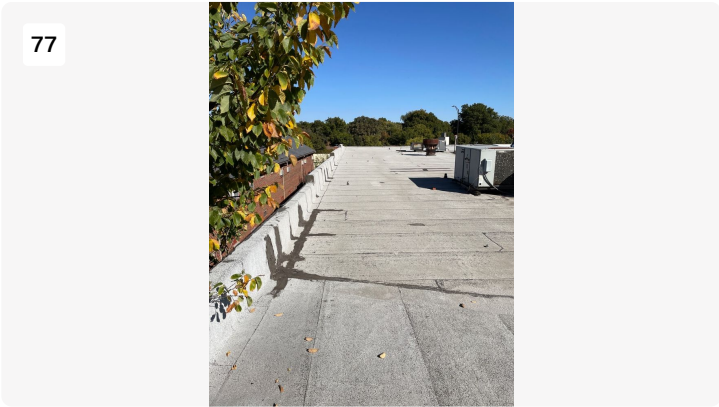
Overview of mod bit roof.
