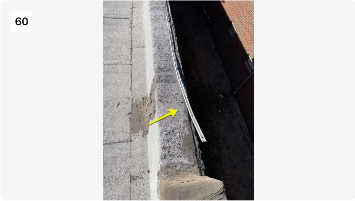
Deficiency: Termination bar no longer fastened to wall.
