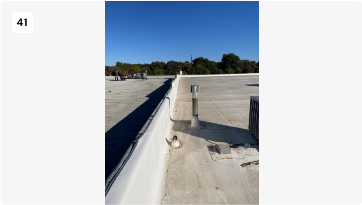
TPO, west wall.
