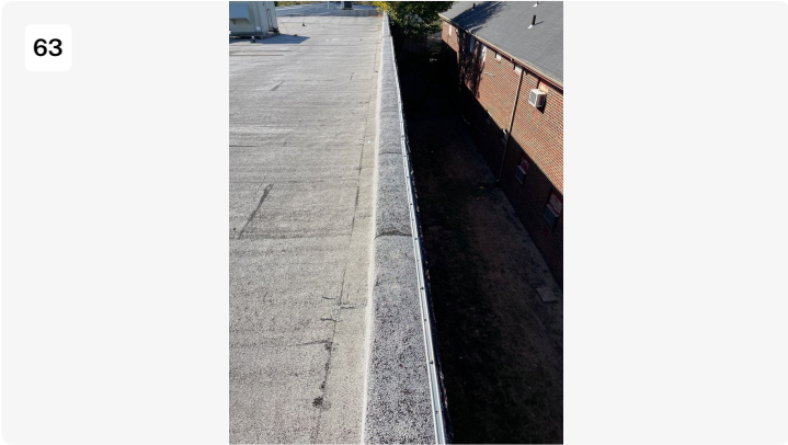
Overview of termination bar.
