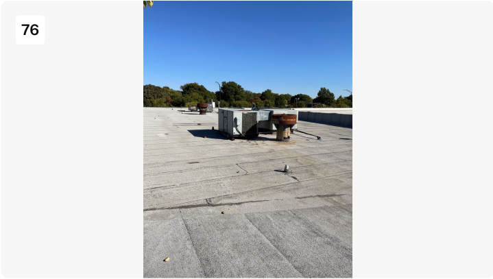
Overview of mod bit roof.
