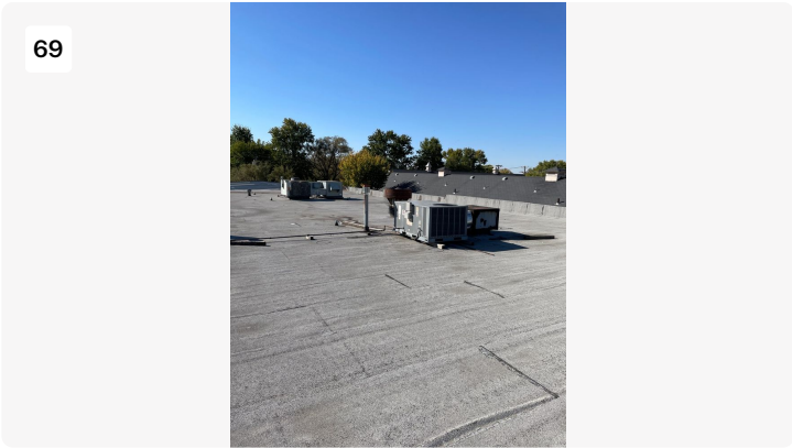
Overview of mod bit roof.
