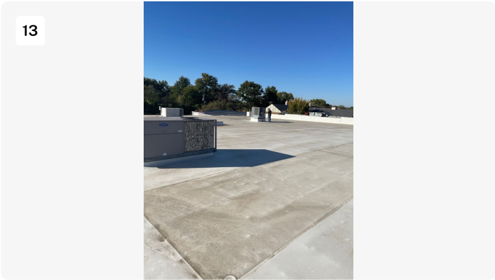
Overview of TPO roof.
