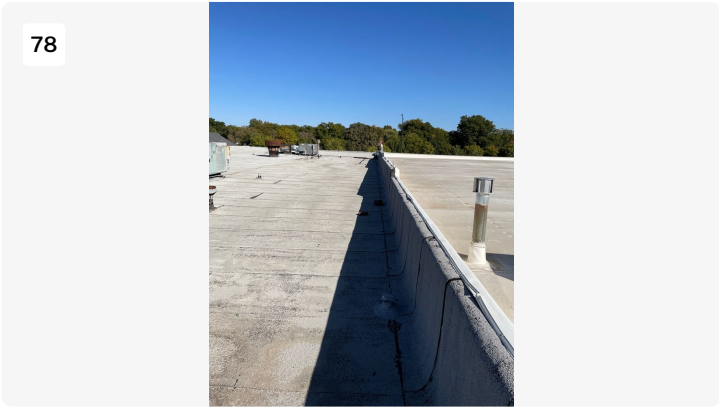
Overview of mod bit roof.
