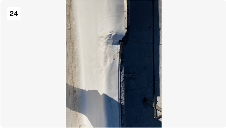
Additional termination bar.
