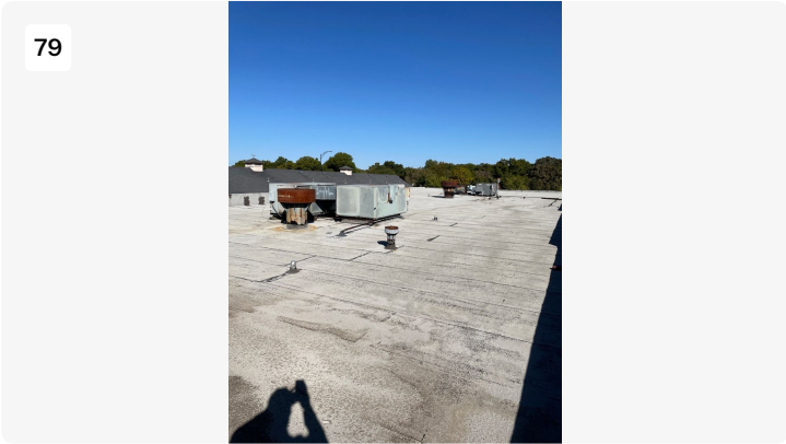
Overview of mod bit roof.
