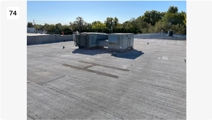
Overview of mod bit roof.
